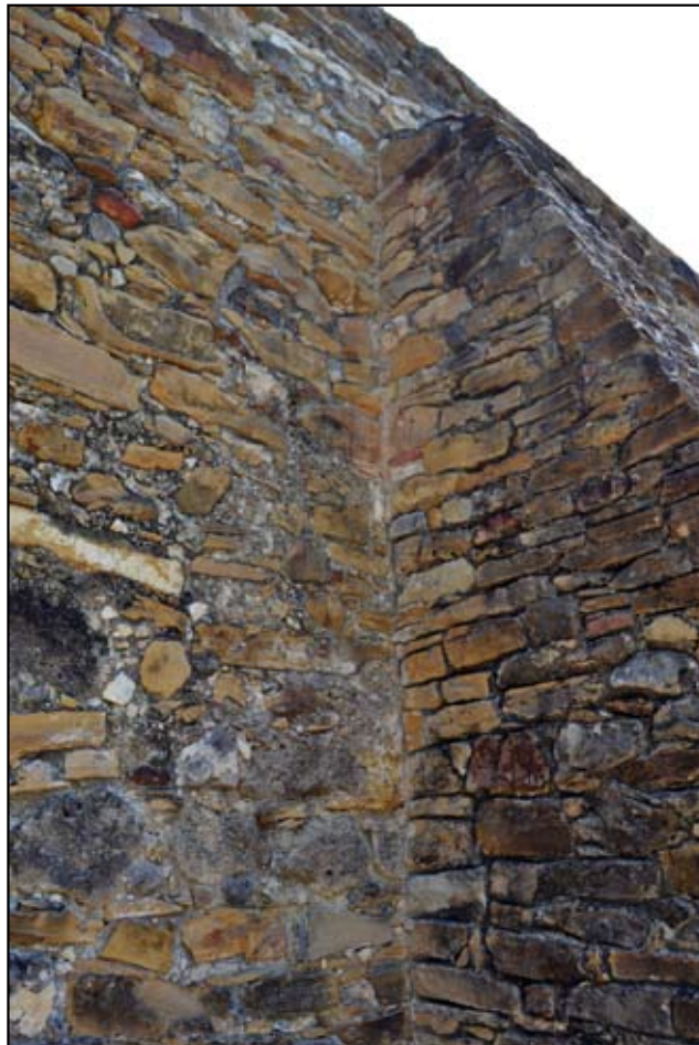
Plate 26. Highly variegated stone [left] mixed with gravely cement in west elevation. Photograph by author.
