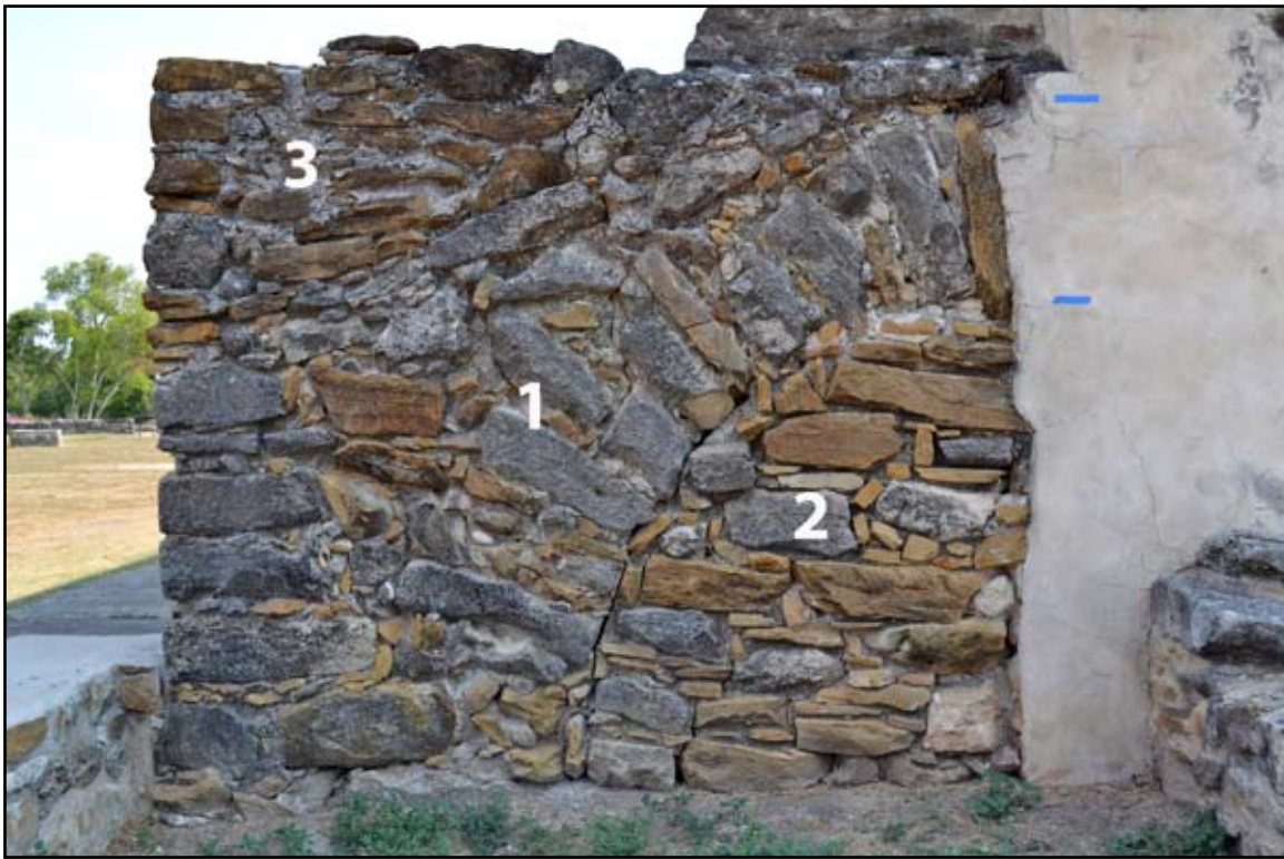
Plate 15. Buttress (1) at northeast corner of chapel that was blocked (2) and squared off (3) for use as a wall. Photograph by author.
