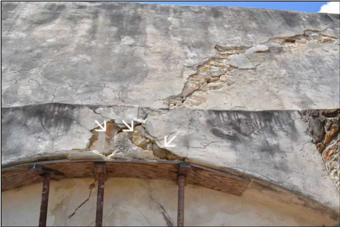
Plate 13. Detail above middle door in east elevation revealing arch masonry. Photograph by author.
