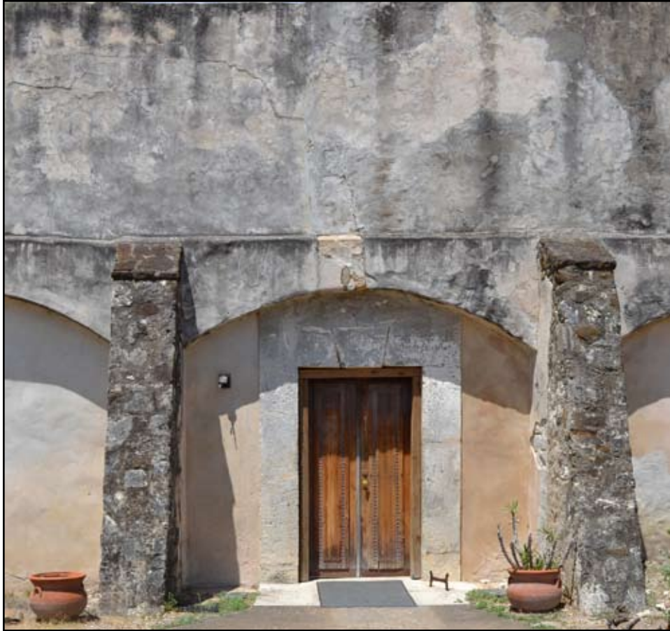
Plate 9. Main entry to the chapel. The C20 stucco cement was stained ca. 1963 and masonry buttresses were added ca. 1968 to several locations along the west and east elevations to provide 'historic' or 'antique' appearances. Photograph by author.
