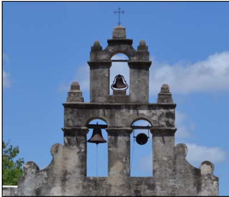
Plate 4. The bell tower is comprised of two tiers of masonry arches now covered with stucco. Photograph by author.
